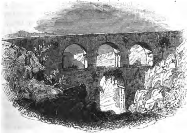
BRIDGE TO THE WEST OF RHITHYMNOS.
