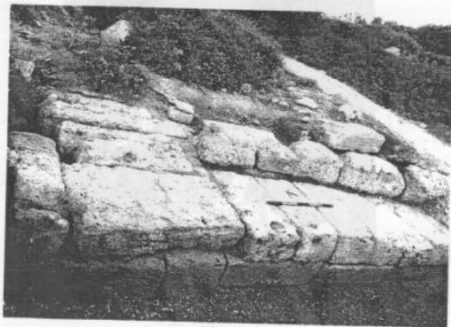
15.7 Photograph of quay in military port.
